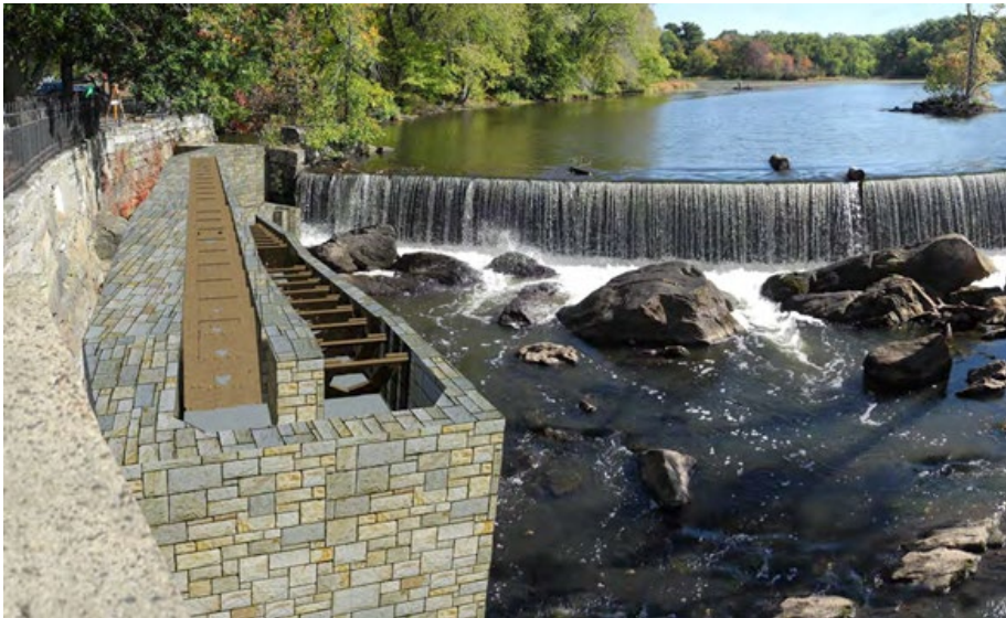
Artist rendering of fish ladder alternative. It is on the 1828 rock ramp to the fishway in the dam which extends upriver. Diadromous Fish Feasibility Final Report, 2016.
